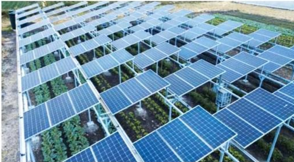
Pictured: Plants being grown in the trial beneath Agrivoltaics. Source: LatiaAgribusinessSol @AgribusinessSol Twitter page.
