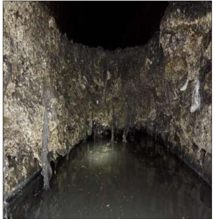
Pictured: The massive fatberg pictured by engineers taken from the Thames Water's Twitter page.
